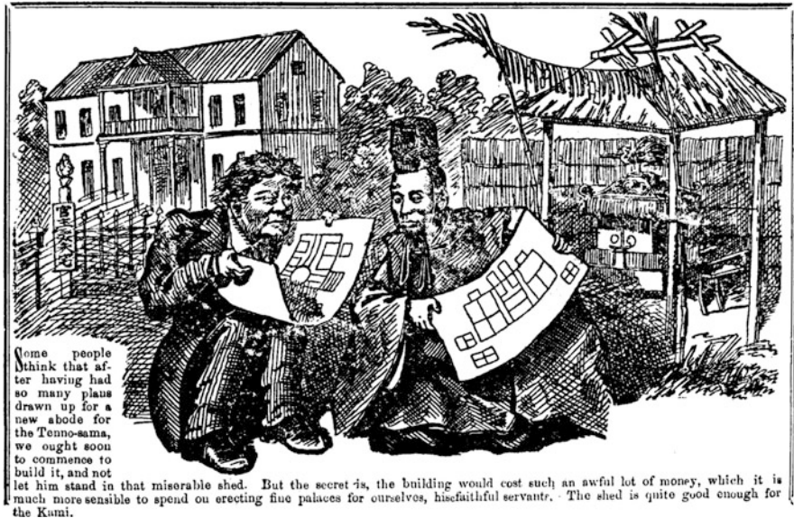
Fig. 12 After the imperial palace burned down in 1873 the government was slow to build a new one. In this cartoon, as two top government officials look at blueprints, one says to the other, 'But the secret is the building would cost such an awful lot of money, which it is much more sensible to spend on erecting fine palaces for ourselves, his faithful servants. The shed (at the background on the right) is quite good enough for the kami (god, i.e. the emperor.)'. Marumaru chinbun 73, 10 August 1878
